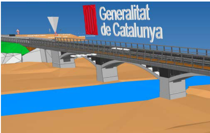
The century-old Cabrianes Bridge over the Llobregat River is being renovated to accommodate additional vehicular, pedestrian, and cyclist traffic.
