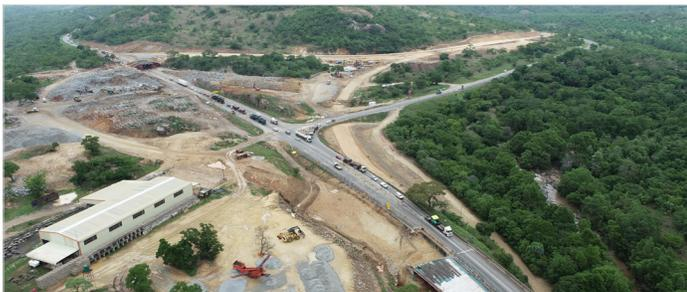
The N4 Montrose Interchange received its first upgrade in over 30 years, replacing an at-grade T-junction with a free-flowing intersection. Image courtesy of SMEC South Africa.
