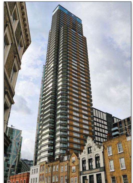
With RAM Concept and PLAXIS, WSP created a more efficient design that reduced both material and labor costs.
